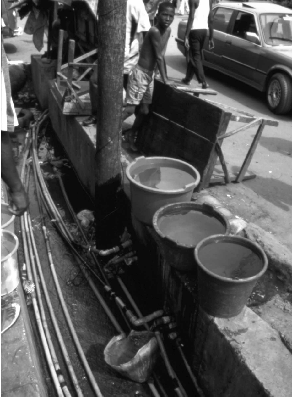
Figure 4. Illegal water connections and street sales of water in Ajegunle, February 2003. Photograph: Matthew Gandy.
